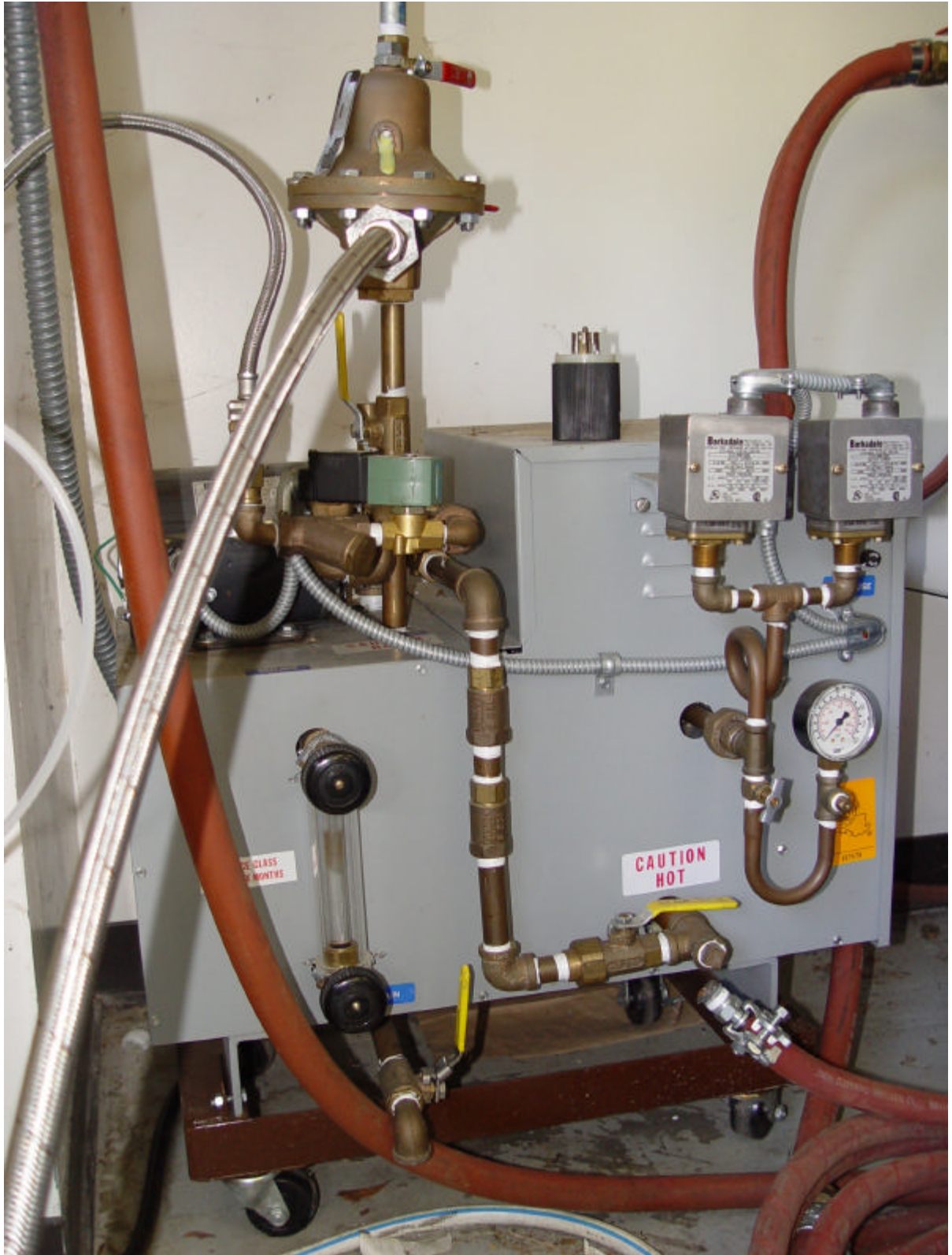
Figure 12. Steam generator.
